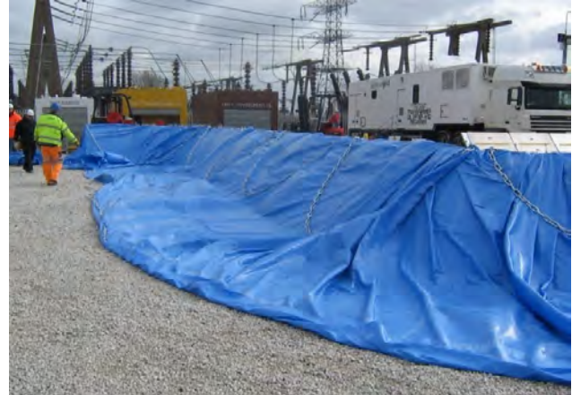
Figure 10.3 Example removable flood barrier use
